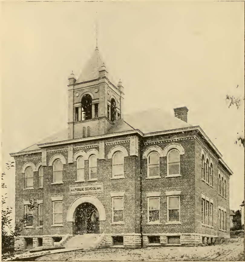
The Fourth School Building.
